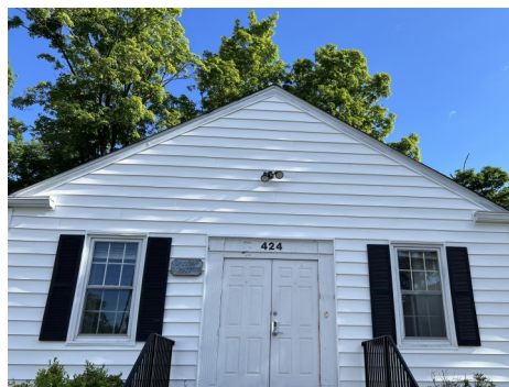
And just like that, Cook Hall has a new façade.
