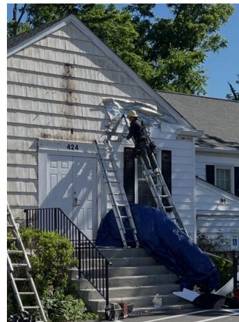
Pujols Roofing and Siding resided the front of Cook Hall.
