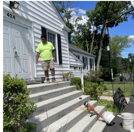
Clem's Ornamental Ironworks replaced the railings.
