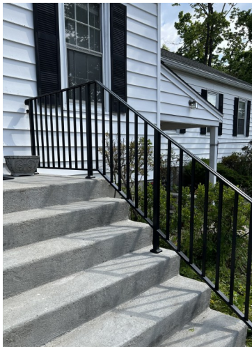
A beautiful job on the railings
