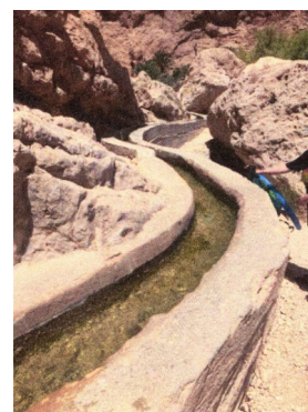
A falaj - a channel that people have been making here since ancient times to irrigate the land.
